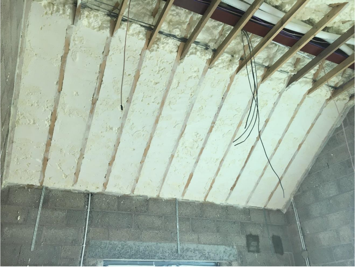
Figure 1 - the Product installed between rafters prior to the application of the plasterboard lining
